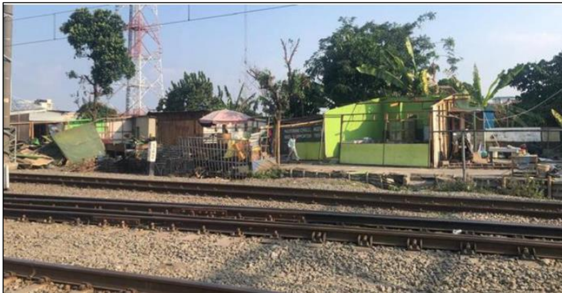
Figure 3. The Condition of the Post-Emptying of Bong Suwung (Source: Researcher Documentation, 2024)
